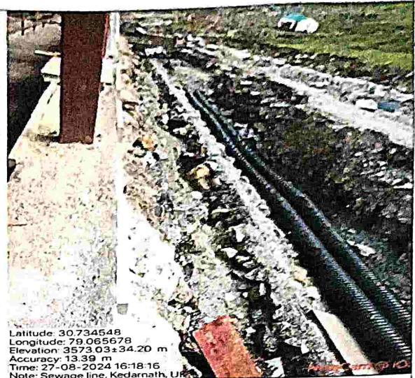
Pic.-6: Construction of sewage lines
