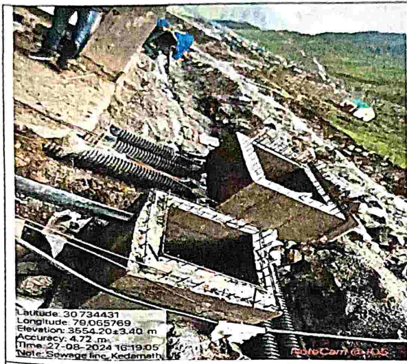
Pic.-5: Construction of sewage lines
