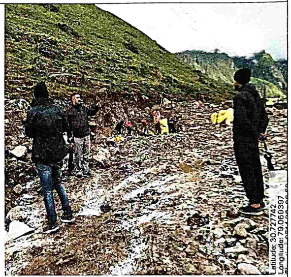
Pic.-12: MSW storage pit
